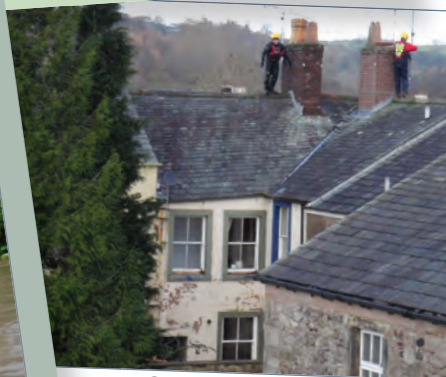
Roof-top rescue service Waterloo Street
