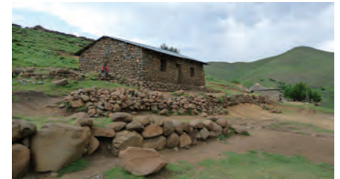
THE EXISTING MALIPHOFU SCHOOL FOR 136 CHILDREN, YEARS 1 TO 6
